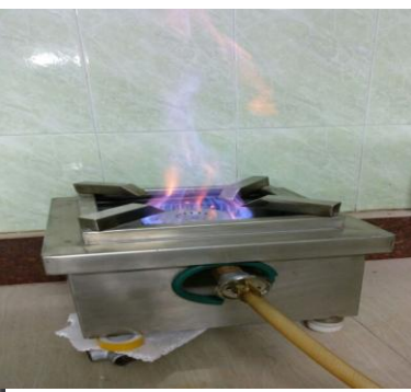
Green temple Bio-gas plant connected with cooking stove
